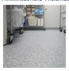
Industrial & Manufacturing facilities Resinous Flooring Systems are well suited for Pharmaceutical Facilities as they provide a durable slip resistant surface and is resilient to harsh environments.
